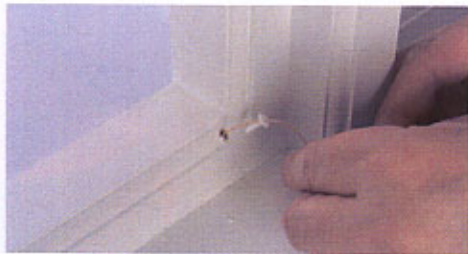
a4. Push cord knot into brass insert, push grommet into brass insert, aligning groove to cord
